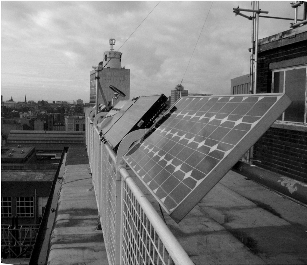
(Fig. 6.3: PV Modules mounted on roof)
